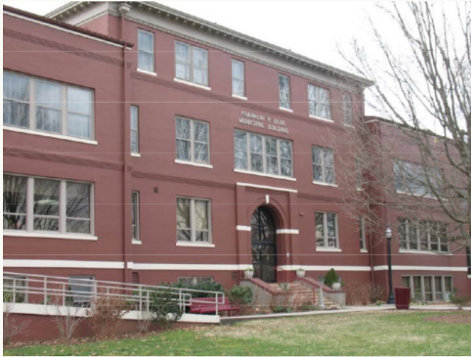
Franklin P. Blue Municipal Building, Warren County
